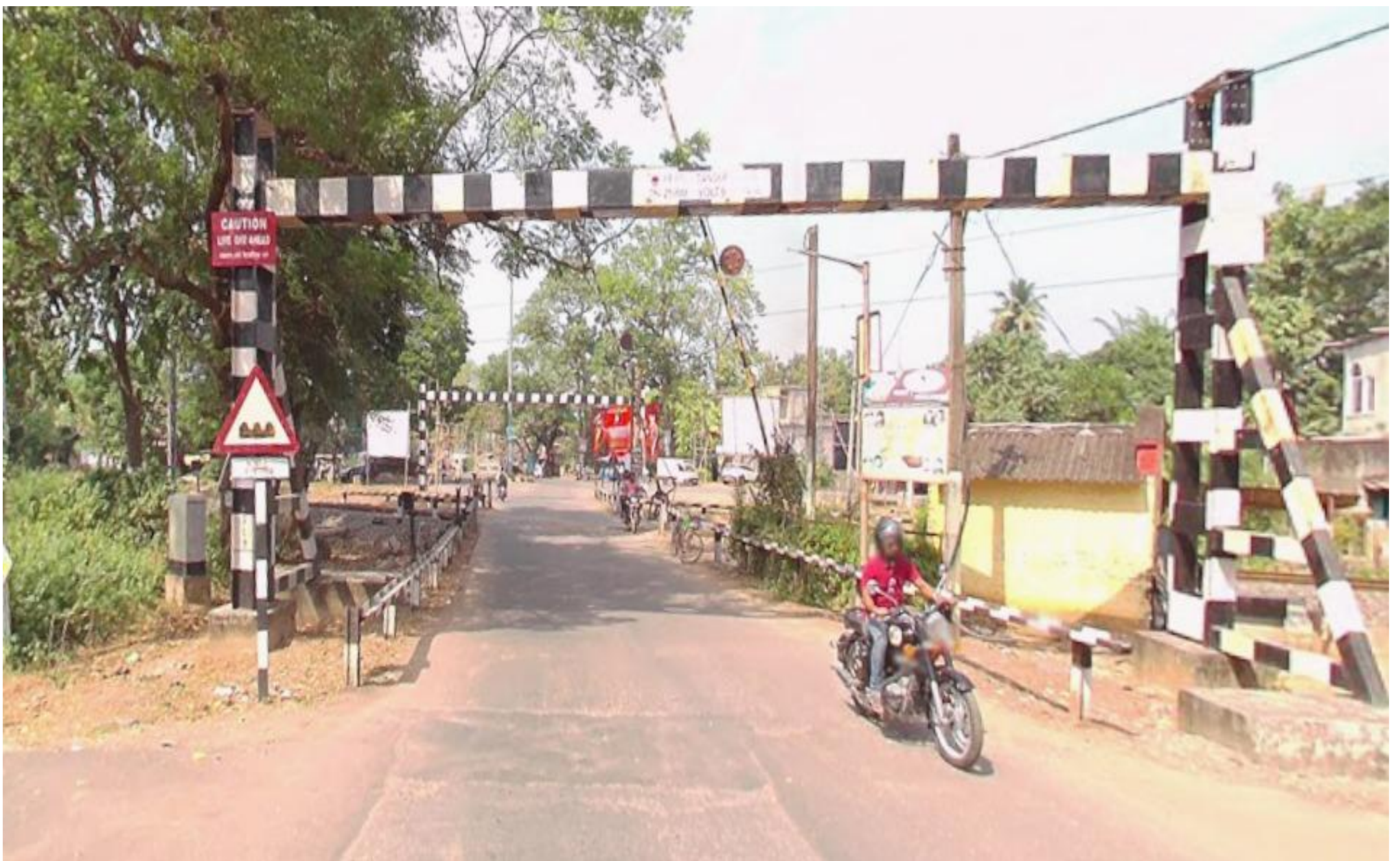
IMAGE: RAILWAY CROSSING ; Risk Level: MEDIUM ; Coordinates: 21.9199201,86.7435814
