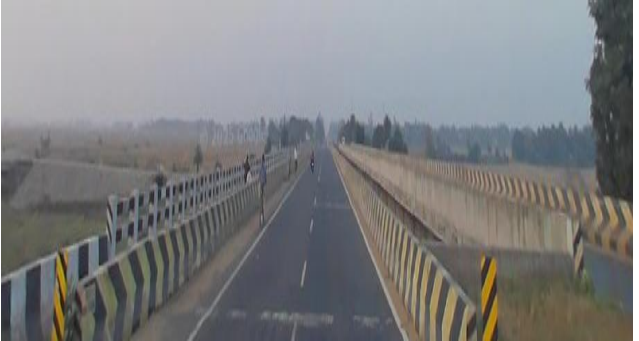
IMAGE: BRIDGE ; Risk Level: MEDIUM ; Coordinates: 21.5810782,86.9292017
