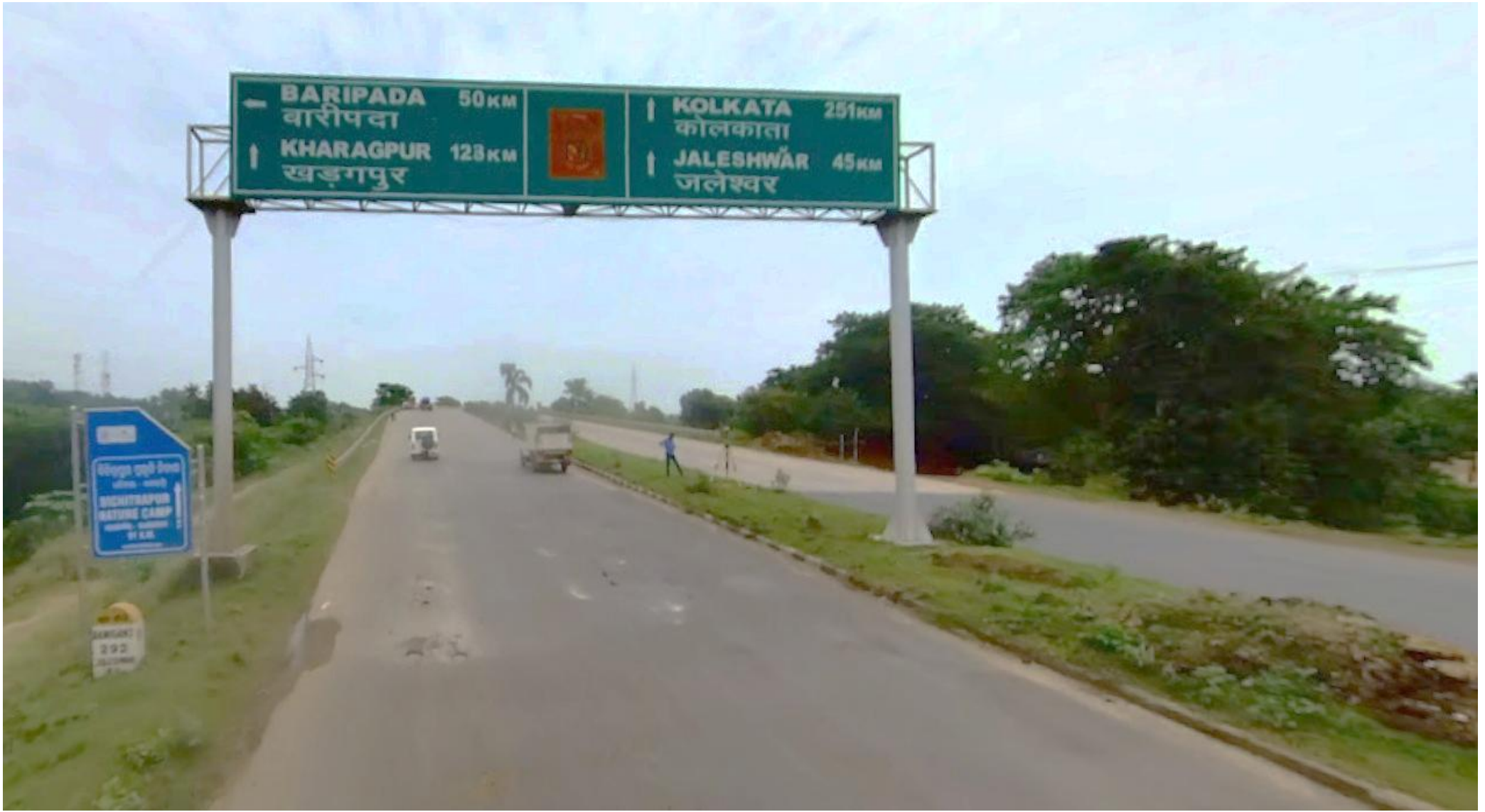
IMAGE: BRIDGE ; Risk Level: MEDIUM ; Coordinates: 21.5500951,86.9218915
